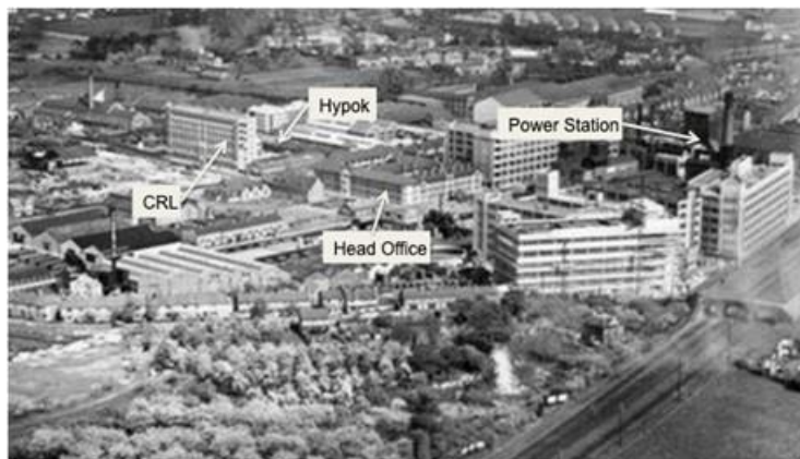
Aerial View of EMI site at Hayes Middx
