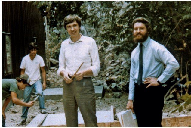
Richard Rzedzian and Ian Pykett, determining the placement of air conditioning units at Advanced NMR Systems, Inc, ca. 1984.
