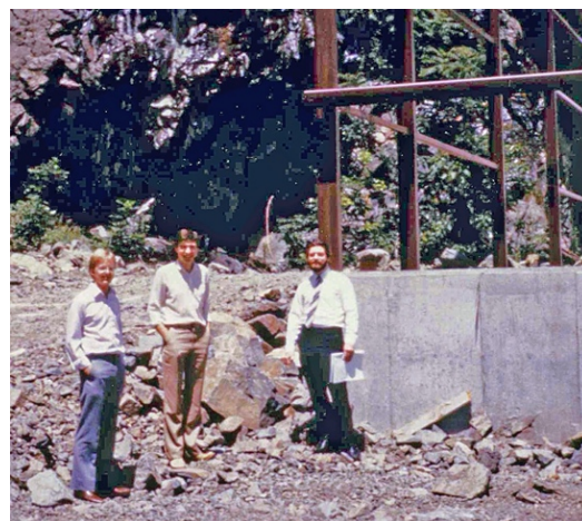
Advanced NMR Systems, Inc's facility, under construction at Sonar Drive, Woburn, MA, ca. 1984. Left to right: Andrew Maudsley, Richard Rzedzian, Ian Pykett.
