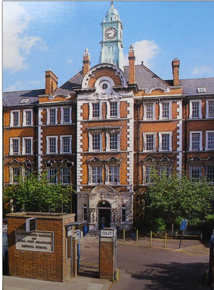
Fig. 27. Hammersmith Hospital (1996). The forecourt from where patients were taken back to Charing Cross Hospital is behind the OUT sign and in front of the entrance to the Hospital.
